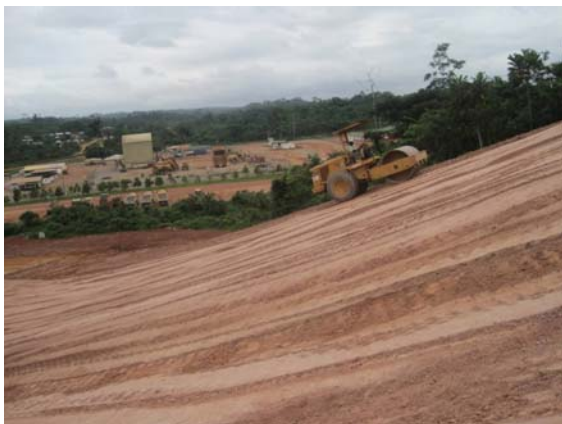
Photo 4 Capping for ARD prevention at Subriso East Waste Dump
