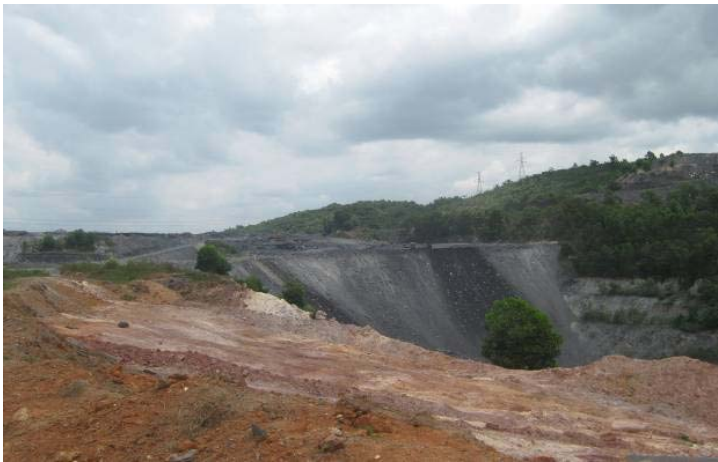
Photo 12 Backfilling the GSBPL Plant North Pit
